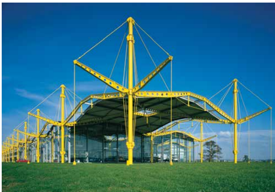
Renault Building, Swindon, UK Архитектор – Foster Associates Подрядчик – Tubeworkers Инженер – Arup
