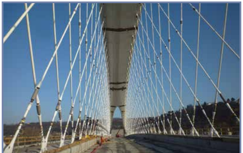
Troja Bridge, Czech Republic Steel Work Designer - Excon Steel Main Contractor - Metrostav
