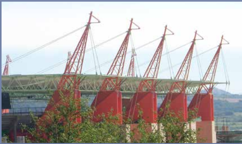
Mbombela Stadium, Nelspruit South Africa Client - Mbombela Local Municipality Structural Engineer - Mott MacDonald
